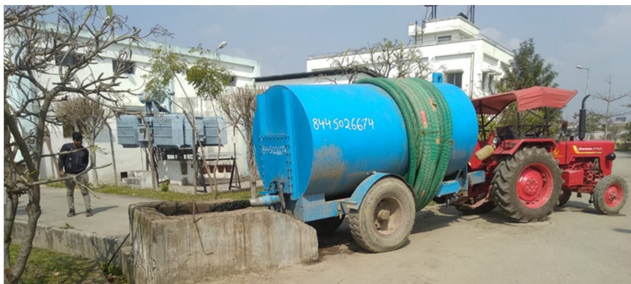
Figure 4: Private vacuum tanker discharging FSS into a chamber connected to MPS in Kargi STP
